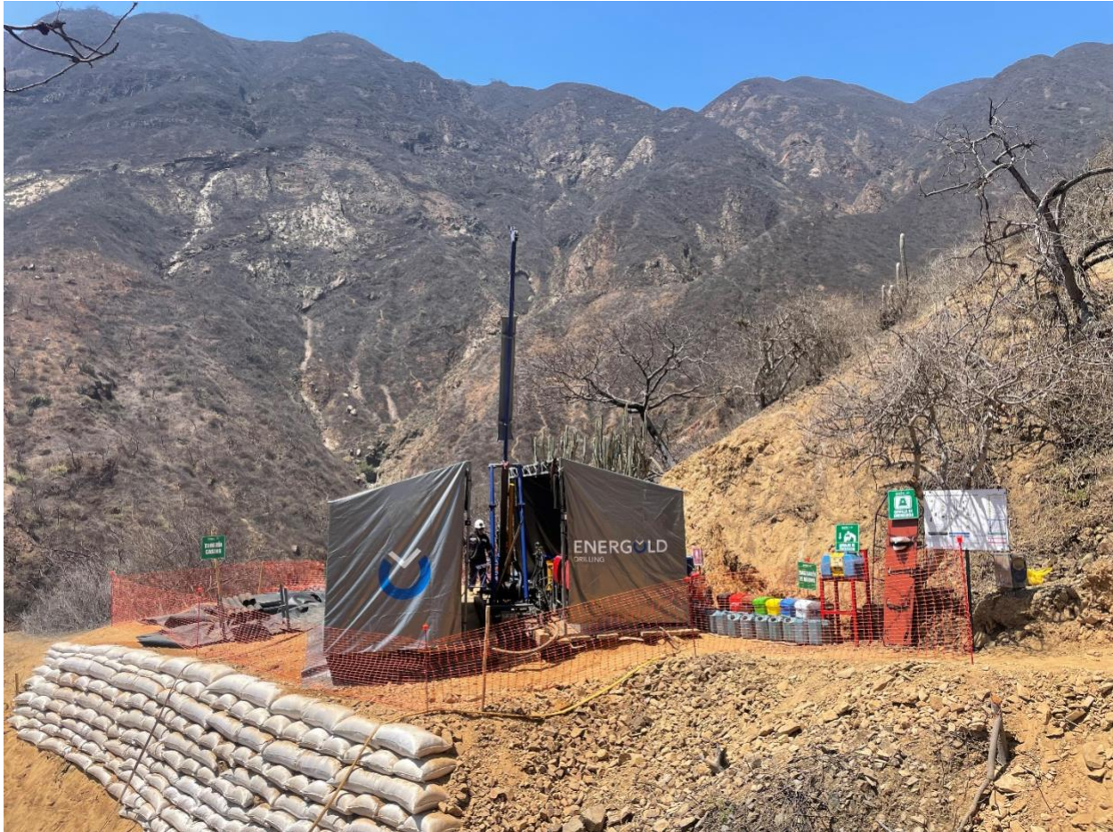
Figure 1: Drill rig positioned and in operation at the Caña Brava Project, Luz Maria porphyry prospect.
